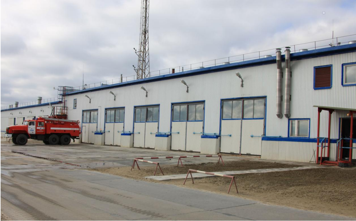
Figure 4. Fire station at production site No. 1
